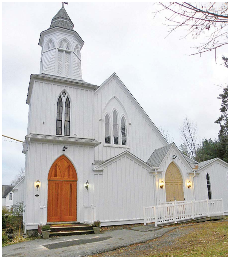
Photo: Welcoming all to worship are the new cedar doors at Holy Trinity. Funding for the doors was in large part a gift from St. Augustine's Church, Conquerall Bank. Photo by Harry Hughes
