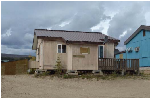
Photo: Bert's new northern home.
