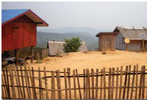
Photo: one of the many latrine construction projects in Laos.
