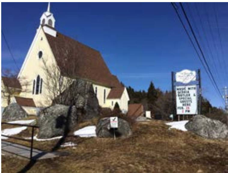
Photo: St James' Church, Boutilier's Point NS
