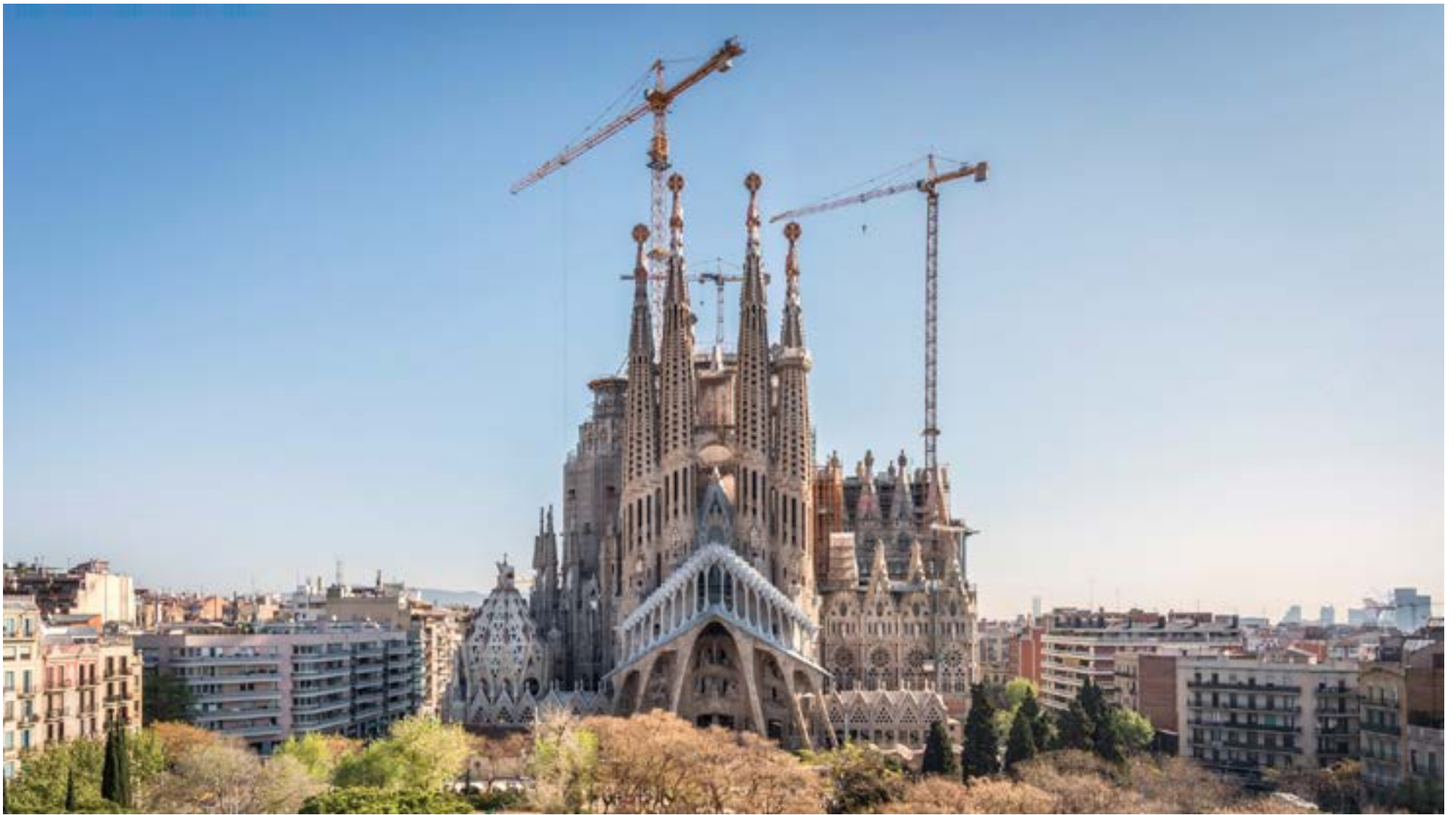
Photo: The Sagrada Familia still under construction. Possible completion date is set for 2028.
