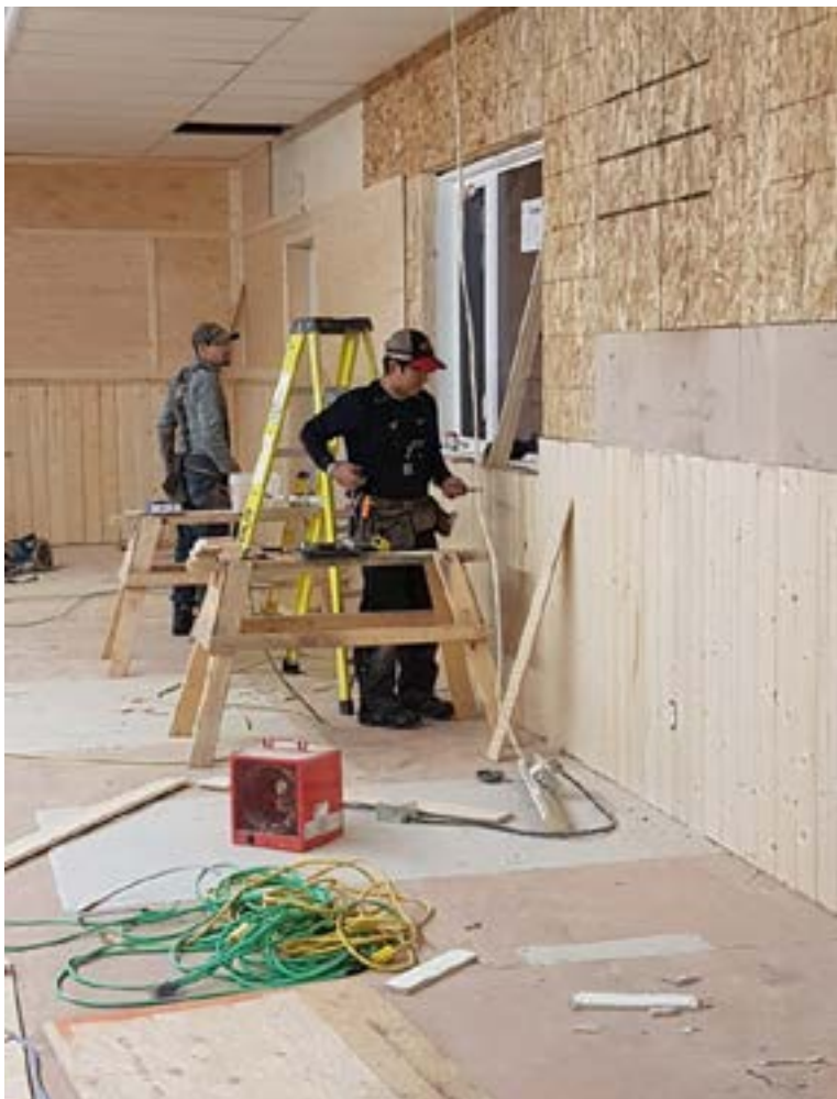
Photo: Renovating the building for a new purpose.
